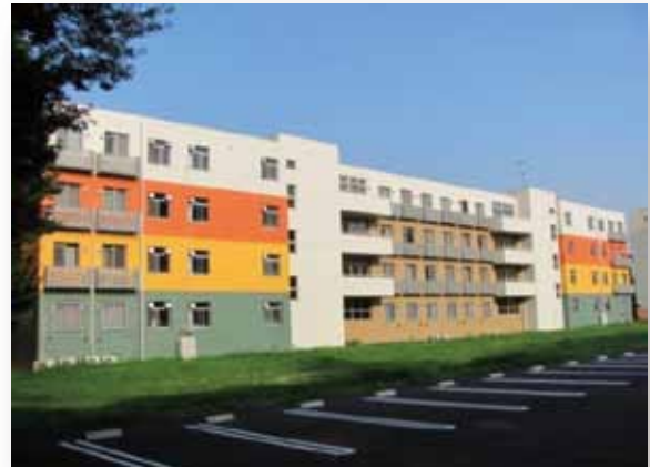
Hirasuna student residence hall after renovation
