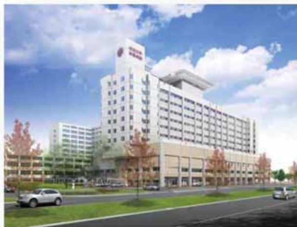
Image of new hospital building exterior
