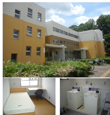
Hirasuna residence hall (after repaired)
